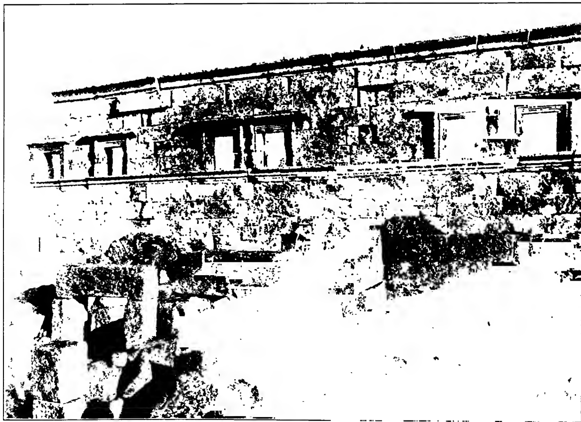
Rear wall of a house at Midjleyyā.
